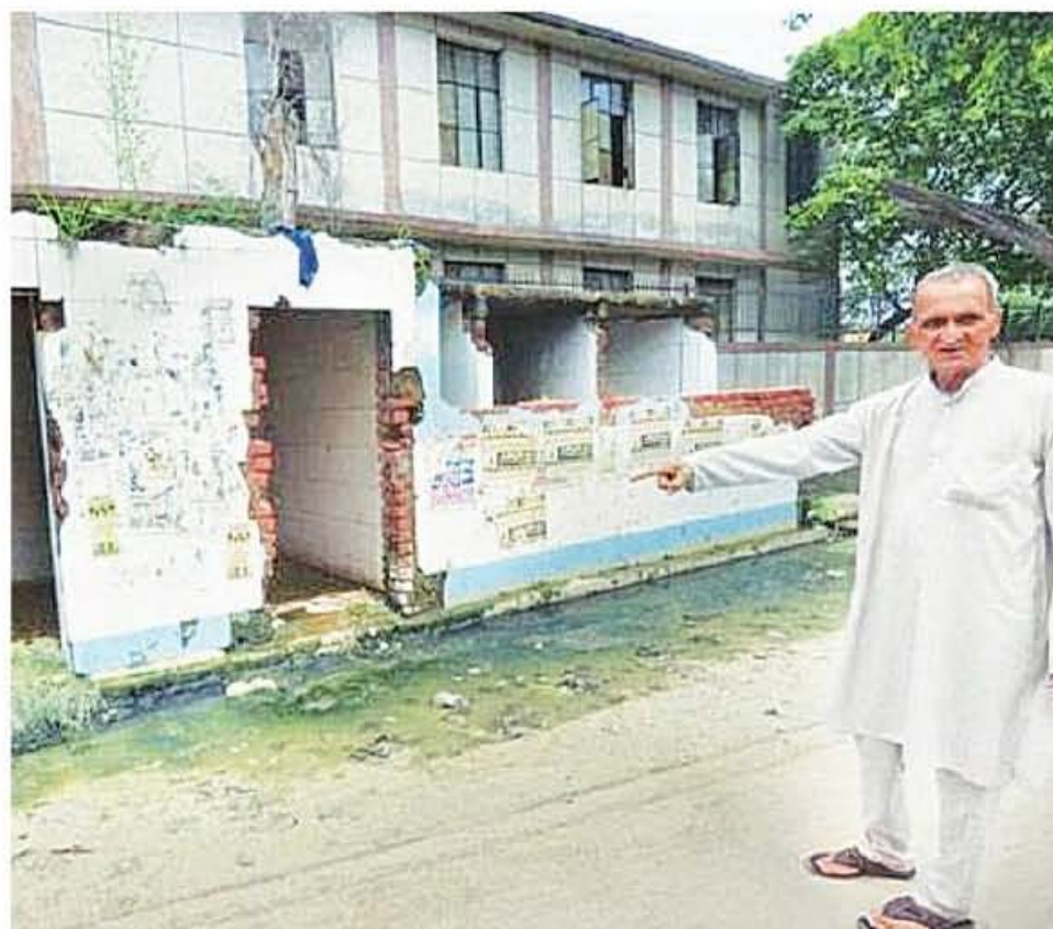
Out of 4,656 community toilets constructed under the mission in the city, most have been constructed by the Delhi Urban Shelter Improvement Board.
